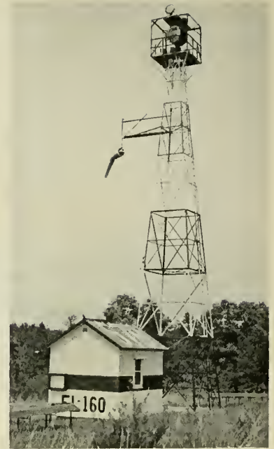
Standard 36" beacon with course lights mounted on top. Wind sock indicates beacon is adjacent to intermediate field
